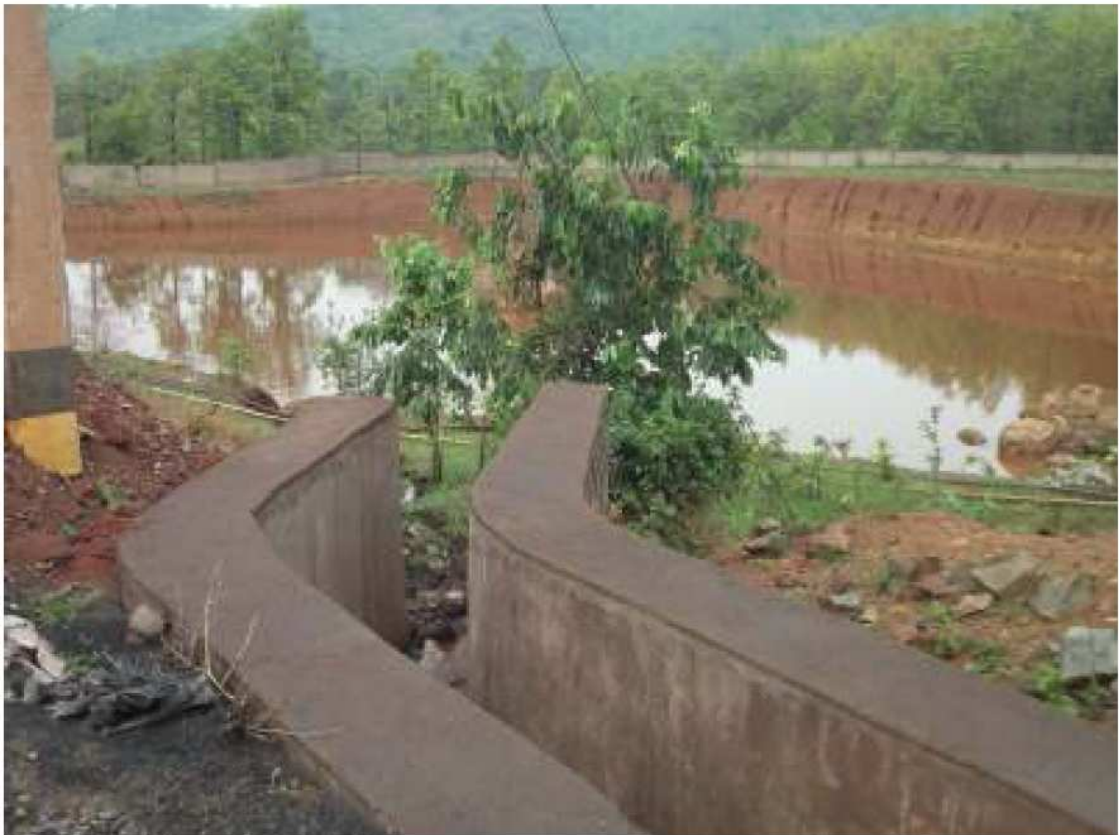
Fig. 5.7: Part of Implemented Drainage Network Connecting Reservoir
