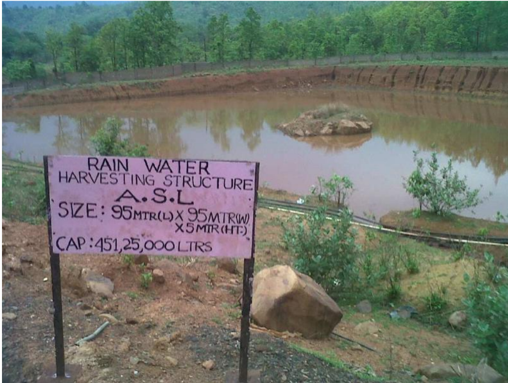
Fig. 5.4: Photograph showing the Implemented Rain Water Harvesting Reservoir
