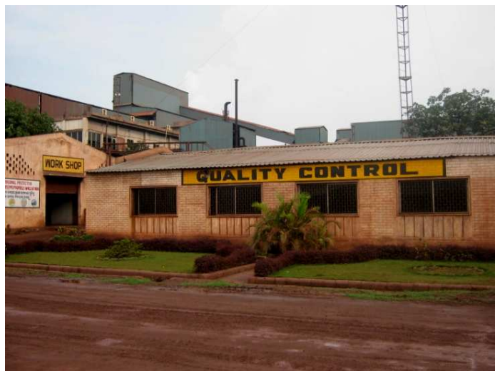
Fig. 5.9: Photograph showing Roof Top Clusters for Proposed Rain Water Harvesting & Artificial Recharge
