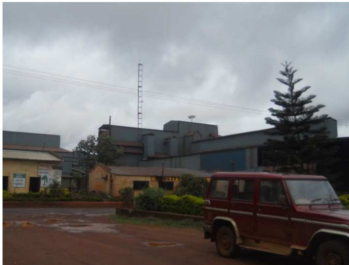
Fig. 5.8: Photograph showing Roof Top Clusters for Proposed Rain Water Harvesting & Artificial Recharge
