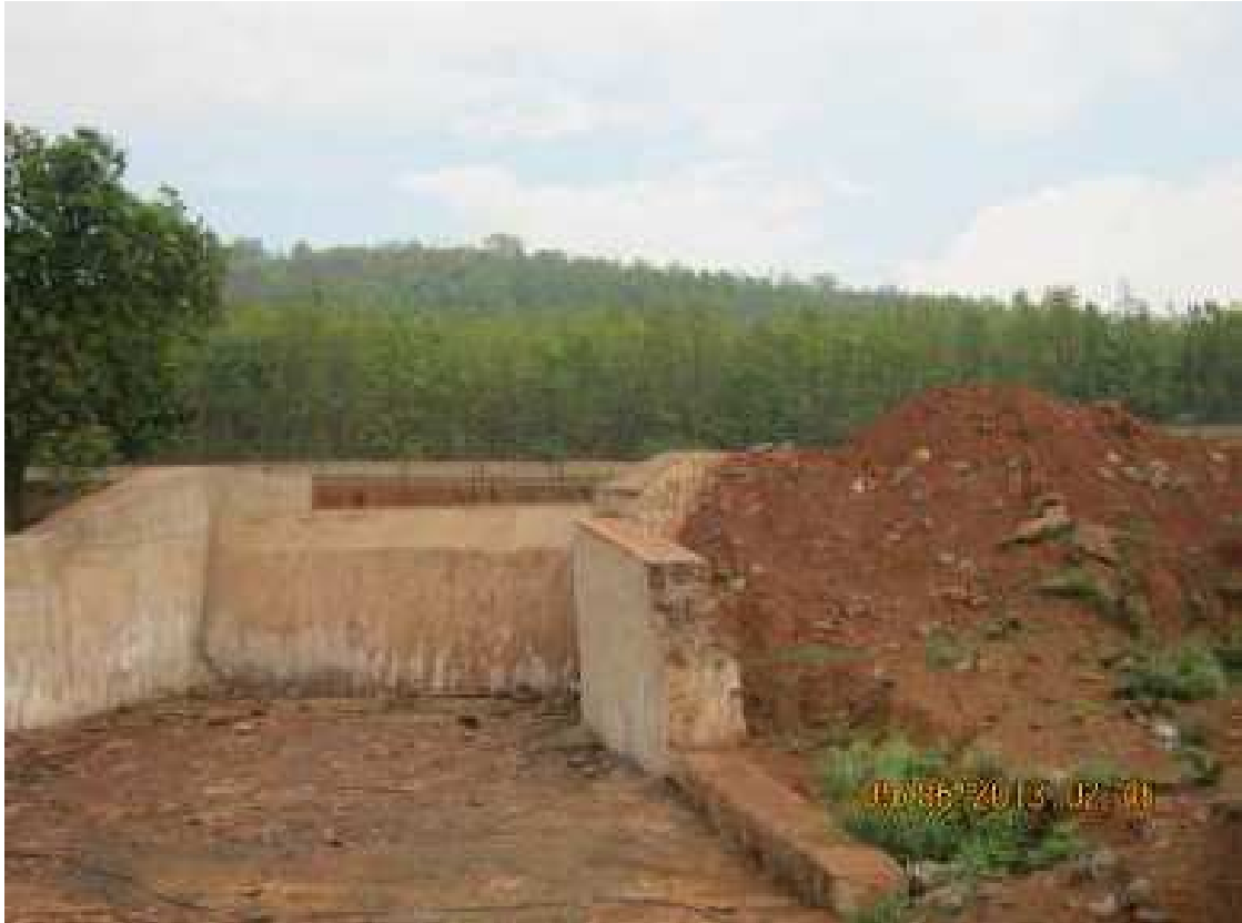
Fig. 5.6: Implemented Check Dam
